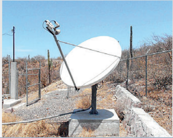
VSAT antenna at auxiliary seismic station AS65, La Paz, Baja California Sur, Mexico, which underwent a maintenance visit in 2013.
