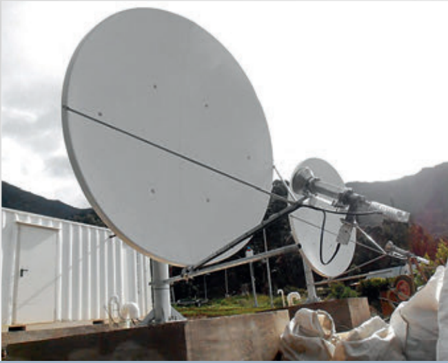
New GCI facility for hydroacoustic station HA3 and infrasound station IS14 in the Juan Fernández Islands, Chile.
