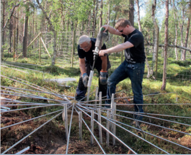
Installing a pipe array at infrasound station IS37, Bardufoss, Norway.
