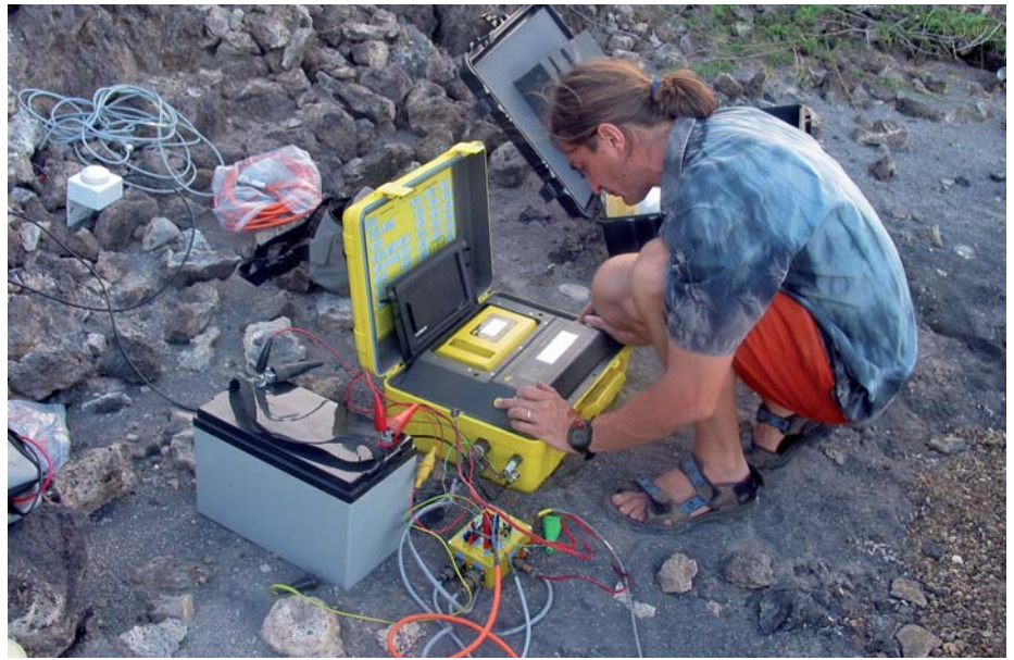
PTS STAFF MEMBER SETTING UP EQUIPMENT FOR NOISE STUDY CLOSE TO THE DIESEL GENERATORS, MARCH 2005, ASCENSION ISLAND
