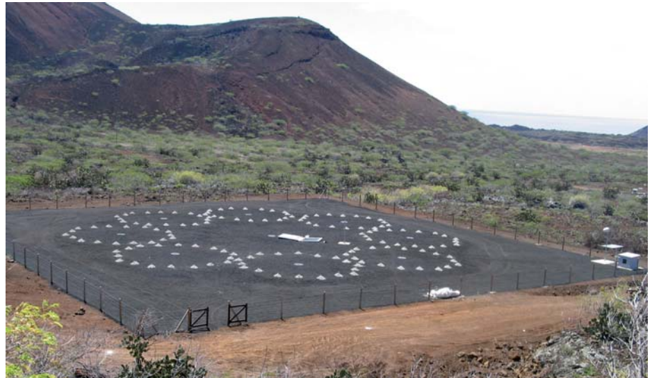
LOW-FREQUENCY INFRASOUND ARRAY ELEMENT, IS50, ASCENSION ISLAND
