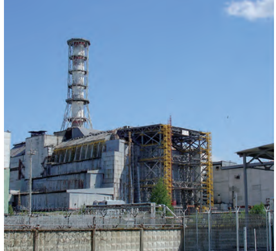
Concrete containment surrounding remains of the nuclear power plant unit in the Chernobyl Exclusion Zone, location of DE07.
